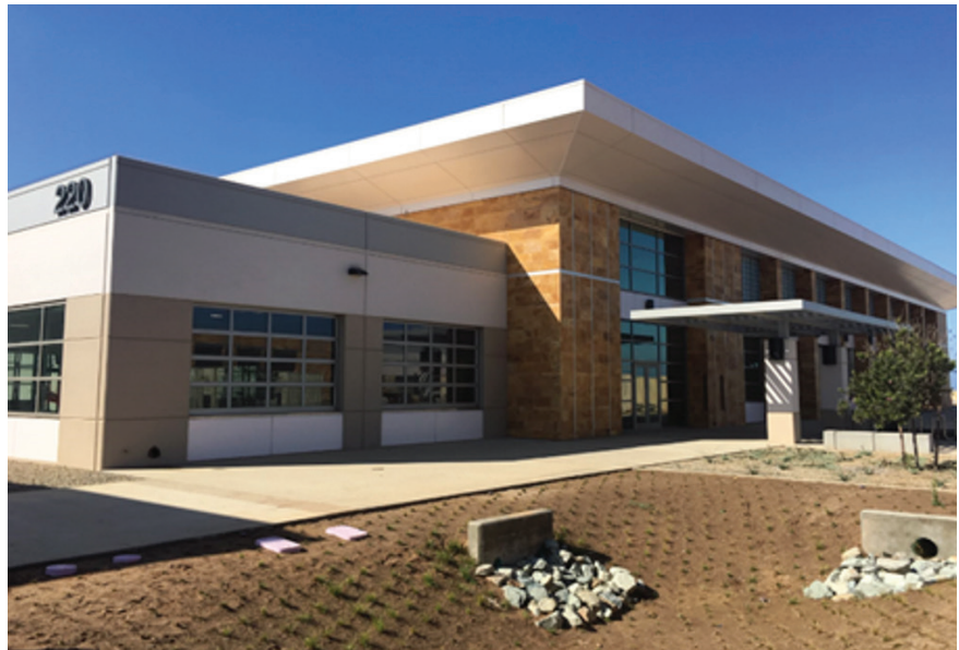
The Silver Strand Training Facility is LEED Silver certified by the U.S. Green Building Council.
